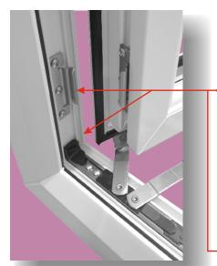
Fit Stay Guard Elite approx 75mm centres from the internal corner as show here. Secure using 4.8 X 25 carbon steel zinc coated screws
